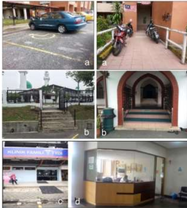
Figure 1: (a) Misused PWDs’ parking and motorcycles are parked along the corridor, (b)No ramp is provided leading to facilities (c) Ramp is provided at the clinic entrance with street furniture (d)the reception counter.
